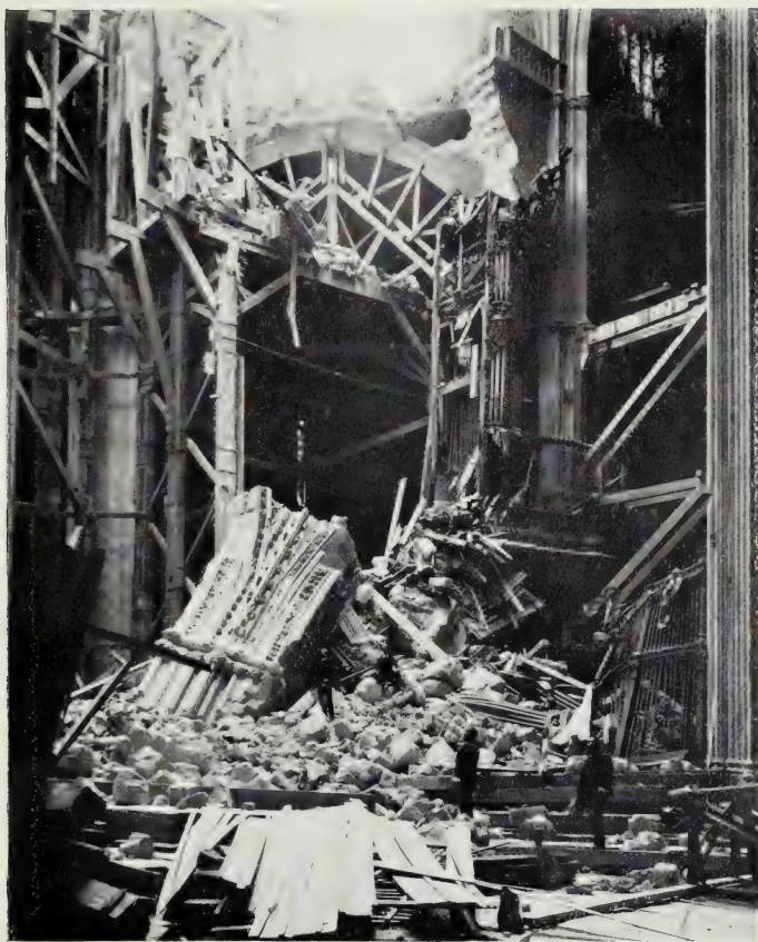
COLLAPSE OF THE CENTRAL VAULTS, SEVILLE CATHEDRAL.
